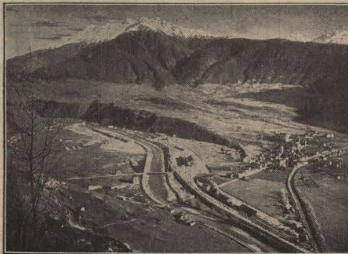
WHERE THE RAILWAY PLUNGES INTO THE BASE OF THE ALPS. Just beyond the station at Brigues the railway line enters the Simplon Tunnel, one of the engineering wonders of the world. The tunnel is the subject of Mr. O. Bolton King's talk to Birmingham schoolchildren this afternoon.
